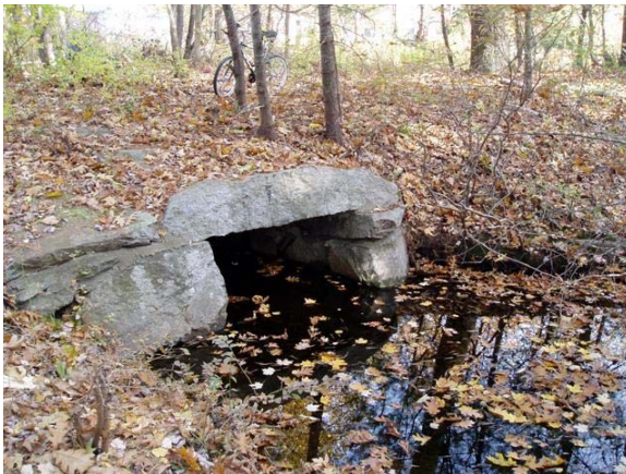
Figure 41: Culvert No. 44.35 South of Old Meetinghouse Road
