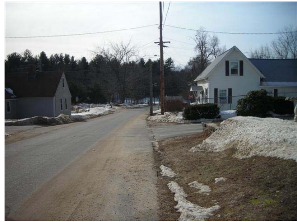
Figure 52: Depot Street Looking West
