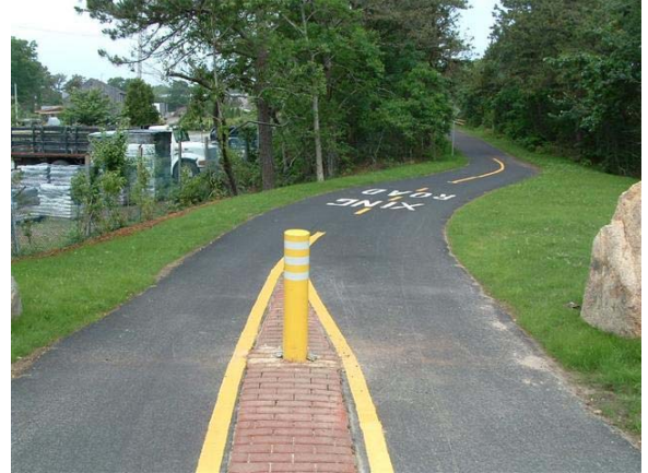
Figure 30: Narrow Median Application
