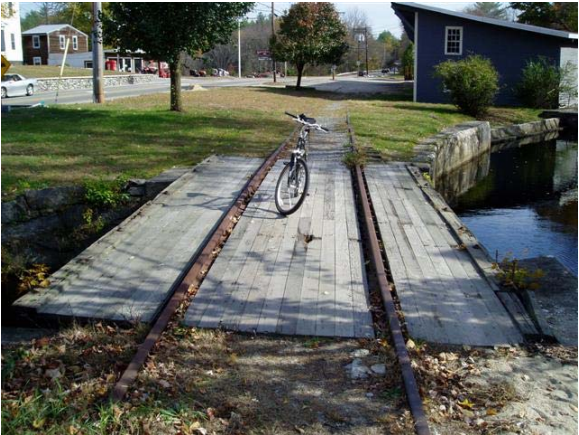
Figure 47: Bridge No. 44.13 Looking South
