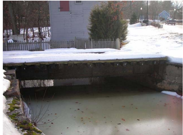
Figure 48: Bridge No. 44.13 Side View
