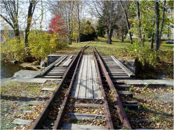
Figure 45: Bridge No. 44.17 Looking North
