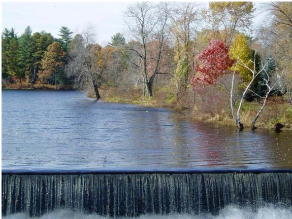
Figure 3: Squannacook River at Harbor Pond
