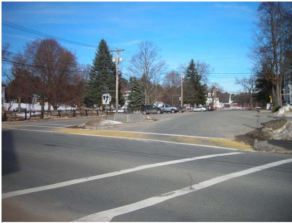
Figure 51: Route 119 Crossing Looking East
