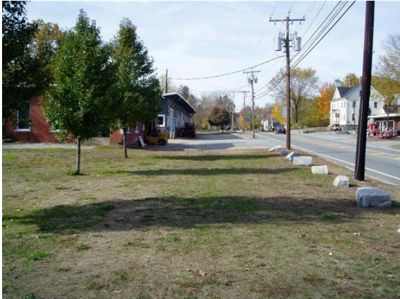
Figure 18: Former Spaulding Leatherboard Factory Site
