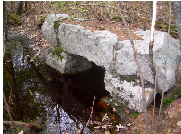
Figure 42: Culvert No. 42.09 North of Crosswinds Drive
