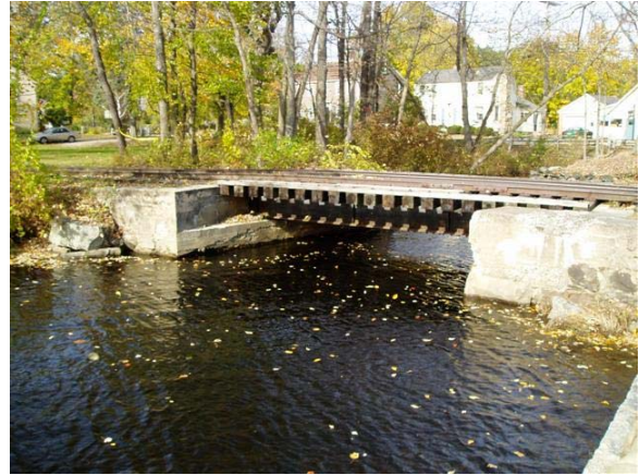
Figure 46: Bridge No. 44.17 Side View
