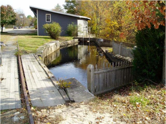
Figure 17: Peterborough and Shirley Railroad Bridge Over Grist Mill Sluiceway
