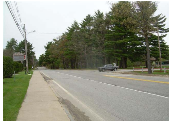
Figure 65: Sidewalk Along Route 119 Looking North From Existing Crosswalk Location
