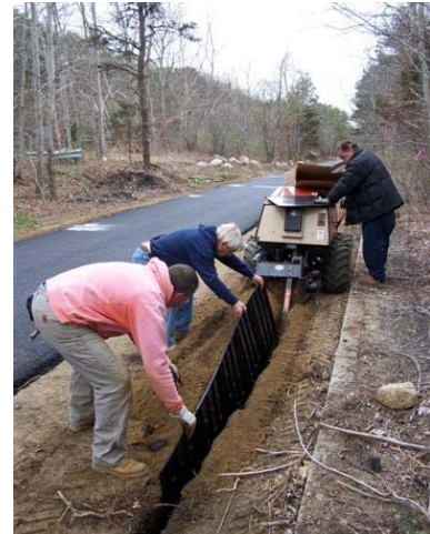
Figure 19: Root Barrier Installation
