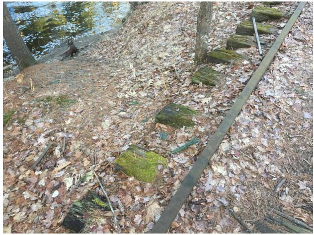
Area 1, Erosional swale leading down to river and undercutting rail bad
